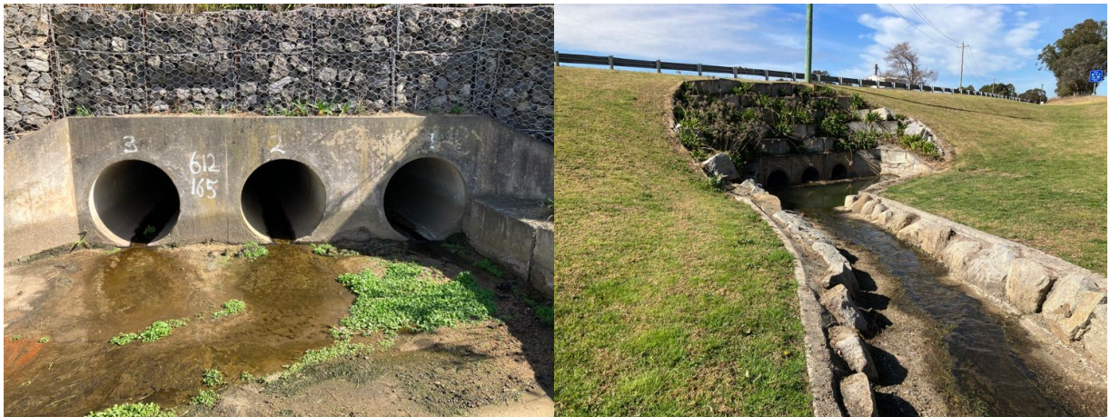
Figure 2-1 Culvert Photographs (Highway inlet left; site inlet, right)
